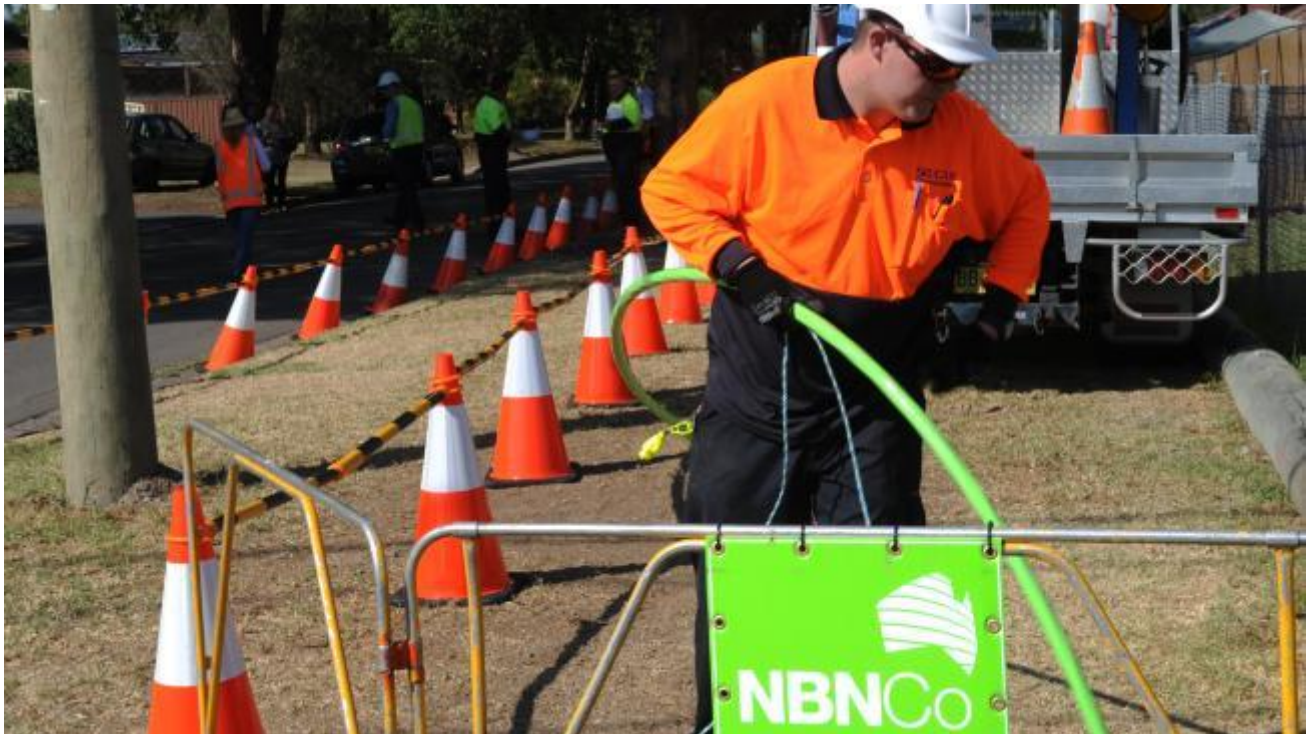
The NBN Co construction team rollout fibre in Penrith.
